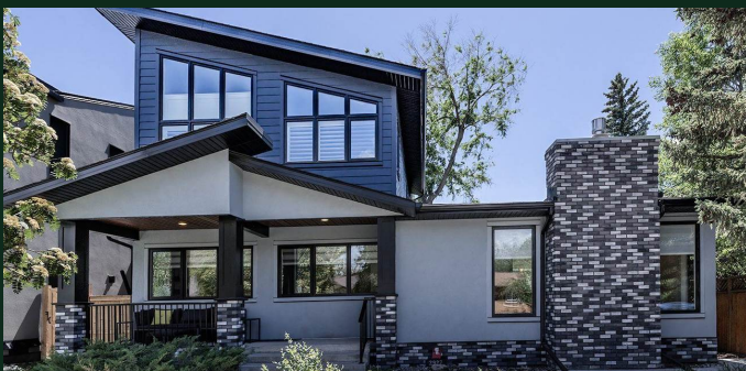
St. Andrews Heights Second-Storey Addition St. Andrews Heights, NW Calgary
