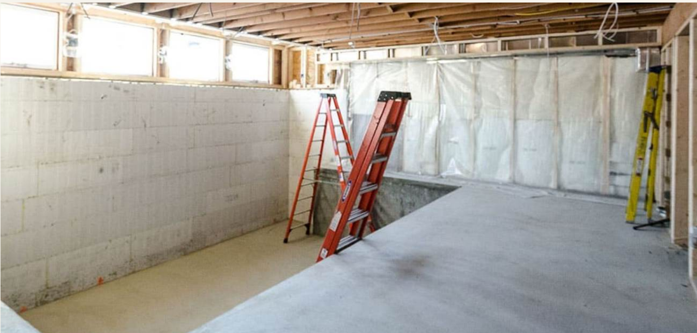
Mayland Heights during construction · what is behind the walls shapes the budget
